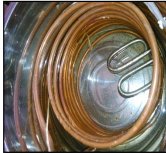
Fig.2.3 Evaporator Tube
